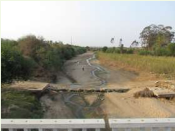
Figure 64: Looking upstream of Sidvokodvo crossing
