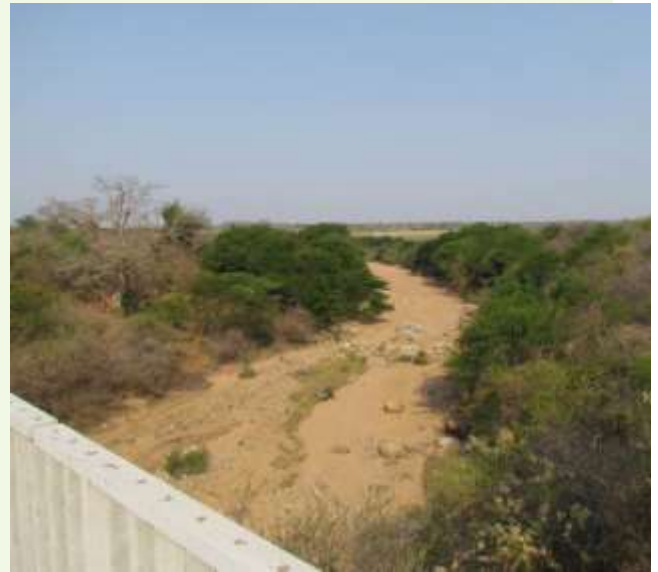
Figure 60: Looking downstream of Mzimneni crossing
