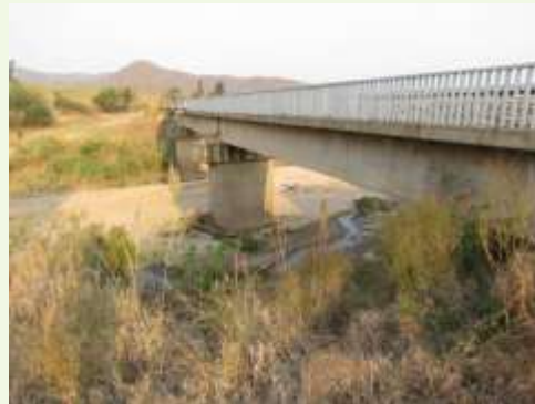
Figure 63: View of Sidvokodvo river crossing
