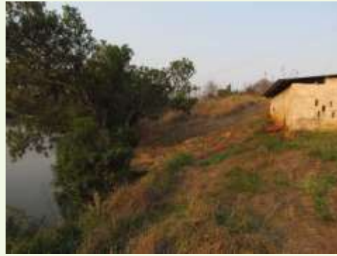
Figure 67: Irrigation water abstraction
