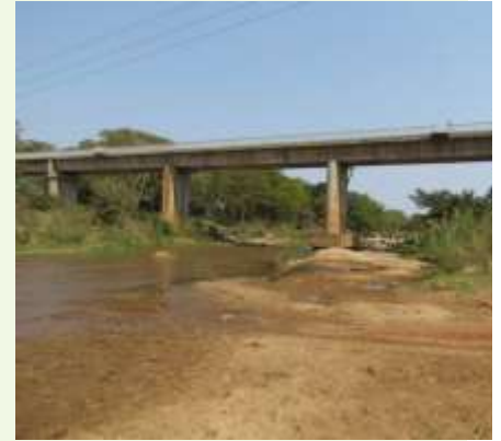
Figure 38: View of Ngwavuma River crossing
