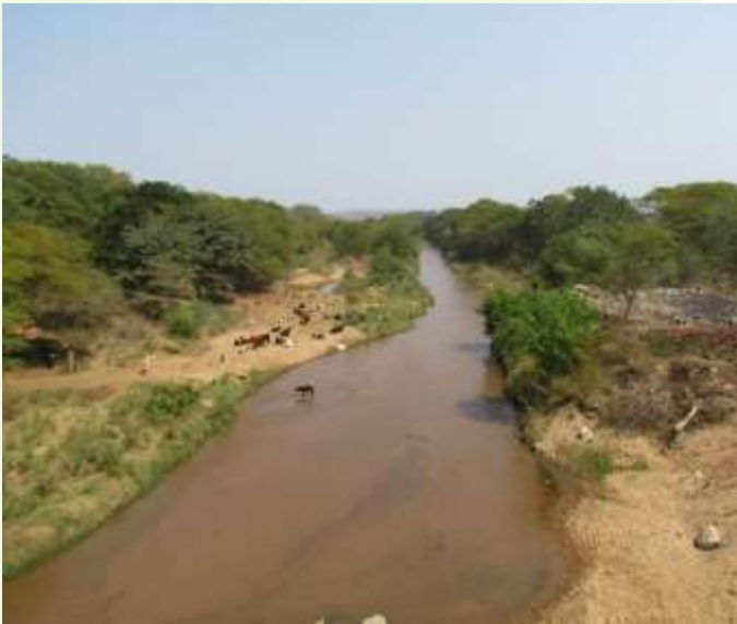
Figure 39: Looking upstream Ngwavuma crossing
