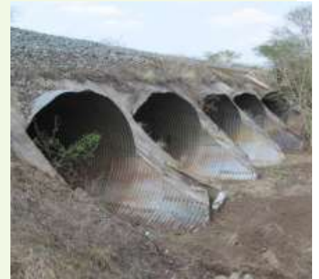
Figure 33: View of Mhlofunga River crossing
