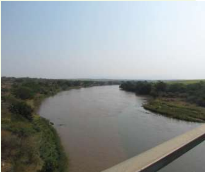
Figure 54: Looking upstream of Usuthu crossing
